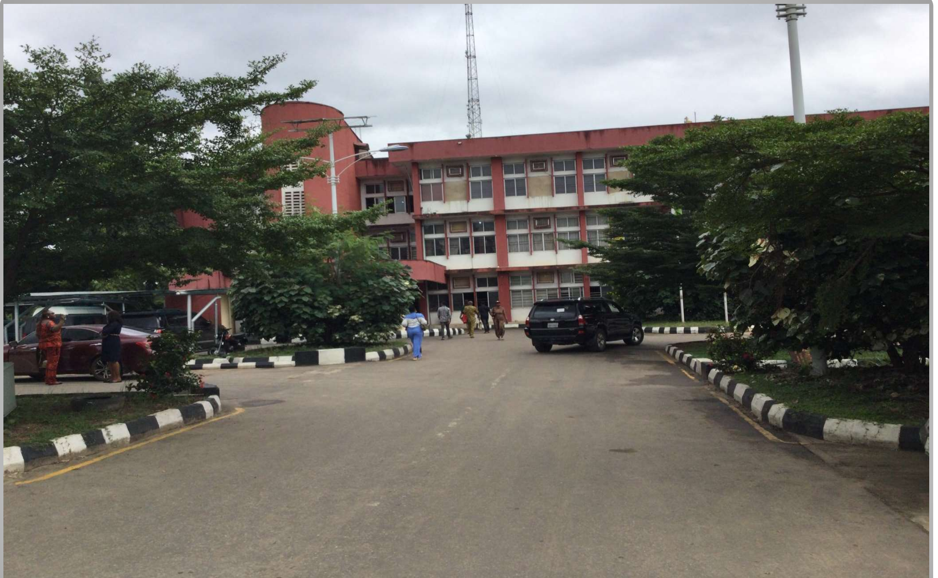
UNIVERSITY ADMINISTRATIVE BUILDING
